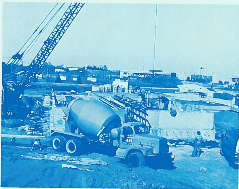
VIDO Building under construction — March 1977.
